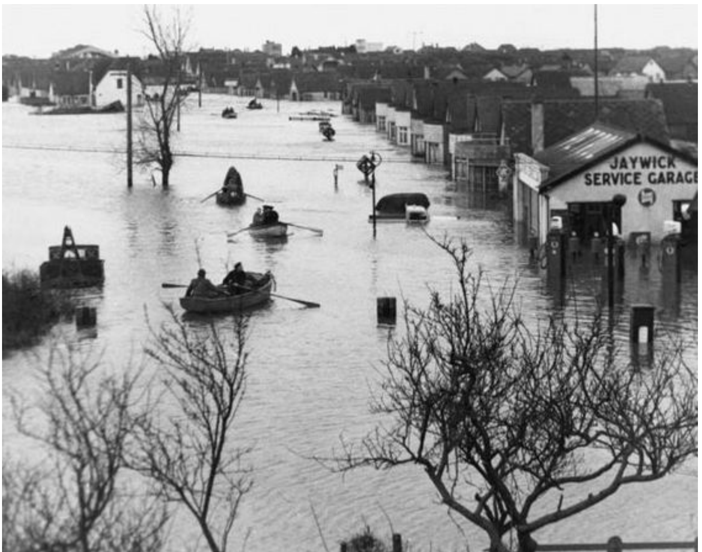
Fig. 64. Photograph of flooding along Golf Green Road in 1953.
