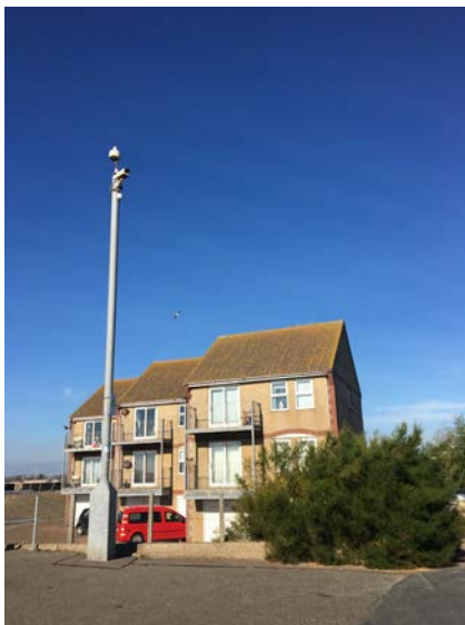
Fig. 53. Newer homes articulated with balconies to reduce visual impact of garages
