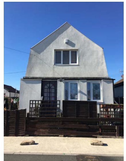
Fig. 54. Mansard/gambrel roof form typical to many Village homes
