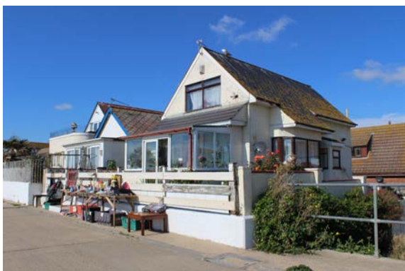
Fig. 55. Seafront home with generous glazing oriented to maximise sea views
