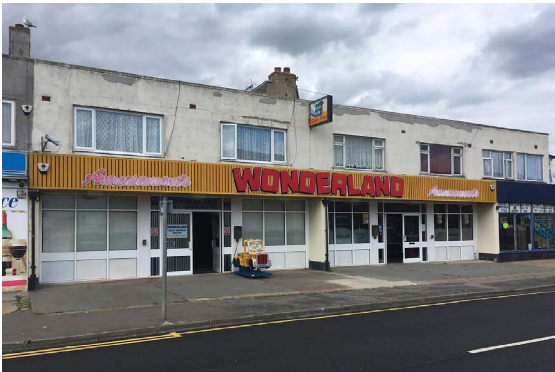
Fig. 38. Former amusement arcade building along Broadway, with flats above.
