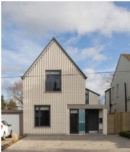
Fig. 57. Gable end to street with room in the roof
